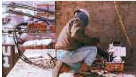
The PE60 used for pre-stressing.
