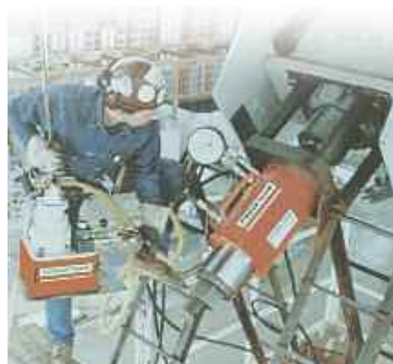
PA554 pump and RH2008 Center Hole cylinder used to tension cables.
